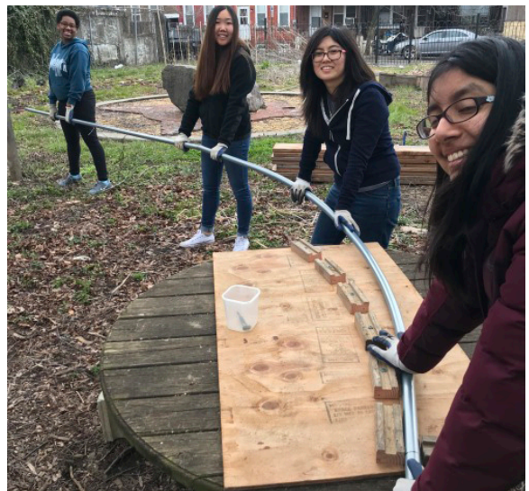
(Top) Sami Khan, G, plants vegetables at Noor Deen Orphan Home in Takengon, Indonesia during his PKG Fellowship. (Bottom) A group of PKG Spring Break students bend metal rods to create a hoop greenhouse in Camden, NJ.
